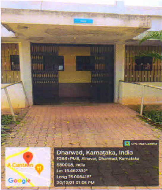
RAMP FOR DIFFERENTLY ABLED STUDENTS
